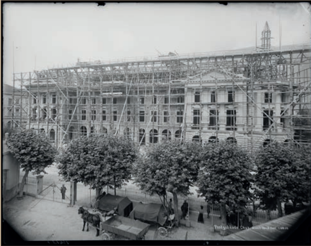
Chur, Baustelle Neue Post (1903) StAGR FN IV 24/30 C 064
