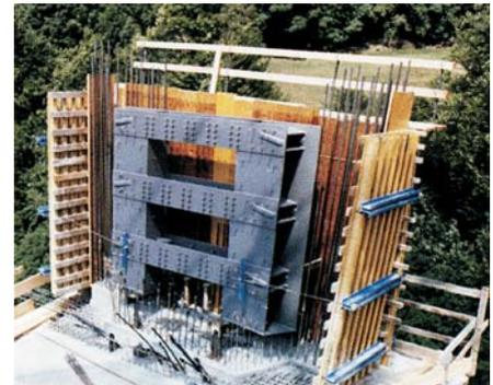
Steel construction for cable anchorage in the pylon formwork
