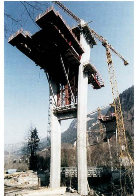
Pier P4 with cantilever construction carriage
