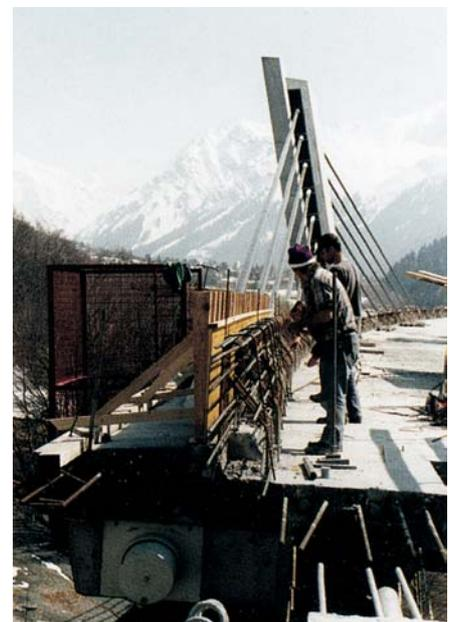
Edge-beam with anchorage and reinforcement of the parapets
