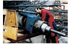
Tightening of the cables with a hydraulic jack
