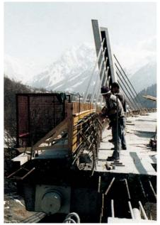
Edge-beam with anchorage and reinforcement of the parapets
