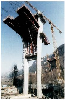
Pier P4 with cantilever construction carriage
