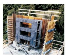
Steel construction for cable anchorage in the pylon formwork
