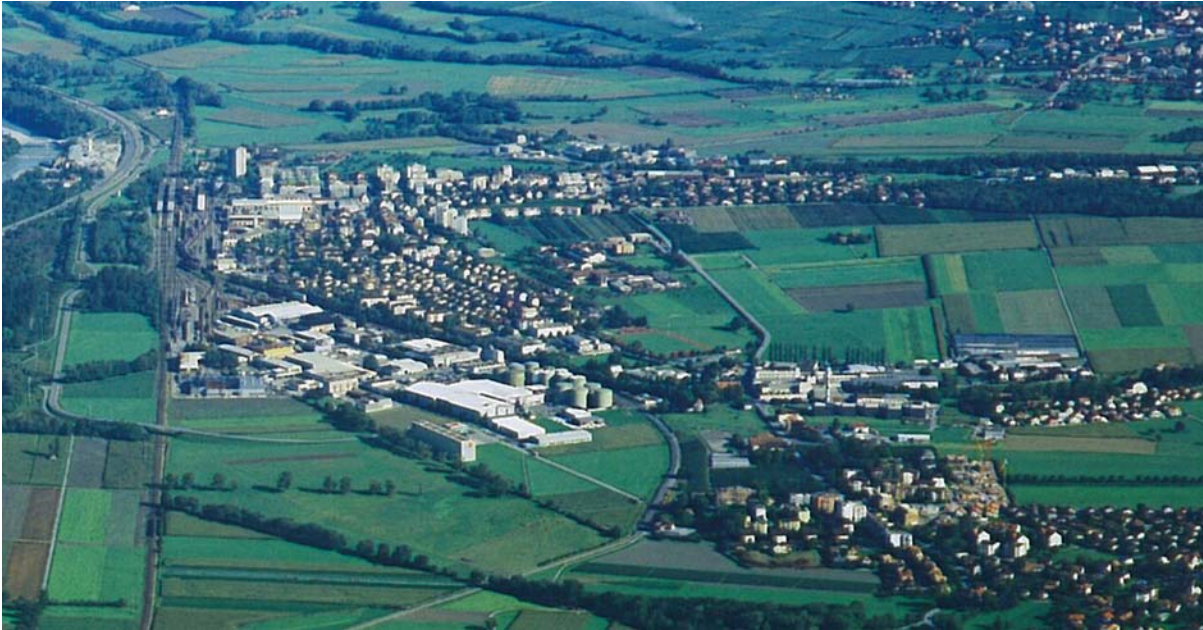
Abb. 2-15 Standort Landquart-Zizers, Luftbild 2006 (Comet Photoshopping GmbH, Zürich)
